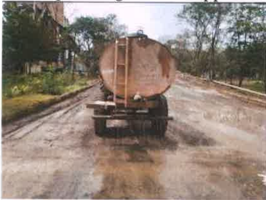
Water sprinkling for dust suppression (Annexure-7)
